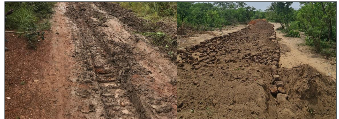
Before Road Repairs
