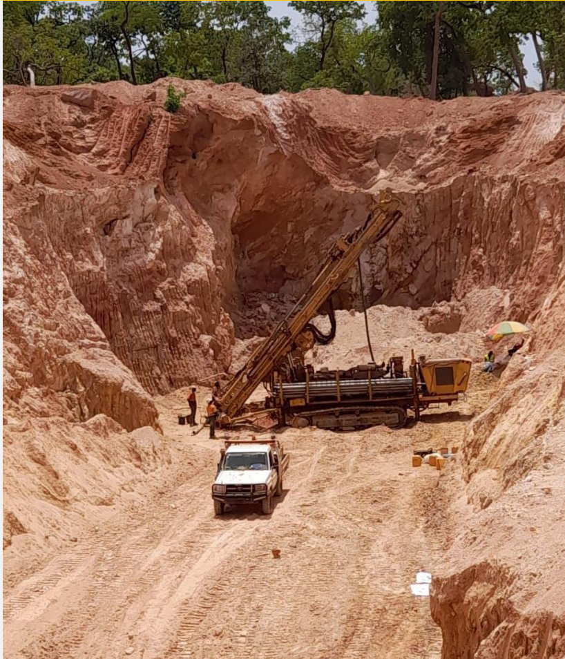
Drill Rig at Mog
